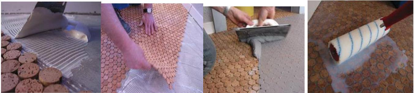
**SUBFLOOR:** Can be installed on concrete, tile backers, or plywood. Concrete must be fully cured and smooth. Surface may need to be etched to enable a solid bond between the adhesive and cork. Plywood needs minimal flex, no less than 1" thick over joists spaced a maximum of 16" on center
