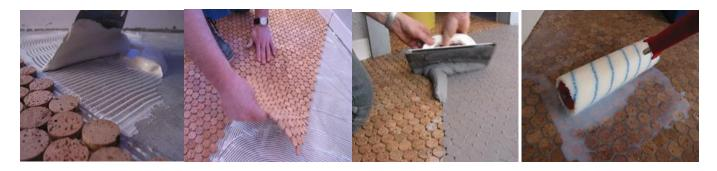
**SUBFLOOR**: Can be installed on concrete, tile backers, or plywood. Concrete must be fully cured and smooth. Surface may need to be etched to enable a solid bond between the adhesive and cork. Plywood needs minimal flex, no less than 1" thick over joists spaced a maximum of 16" on center
