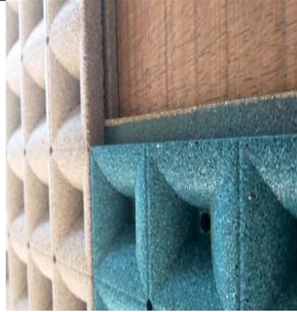
If you do not end on a full piece, cut off the last panel of carefully measure to ensure all panels line up and the edge the row as it is shown in the picture, making sure to detail is as planned.
