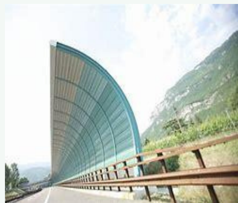
Here is a highway noise barrier.
